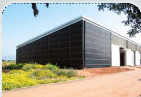
FIGURE 22: Stainless steel panels used to generate process heat in an aromatic-herb drying plant on Mallorca Island, Spain (Photo: energie-solaire.com)
