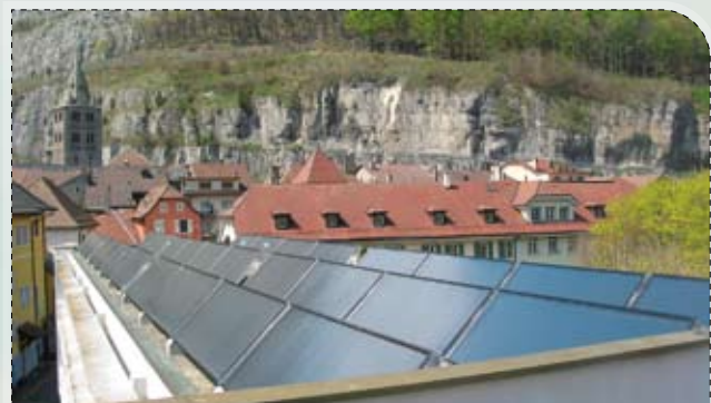
FIGURE 15: Glazed panels are most efficient when oriented towards the midday sun (Photo: energie-solaire.com)
