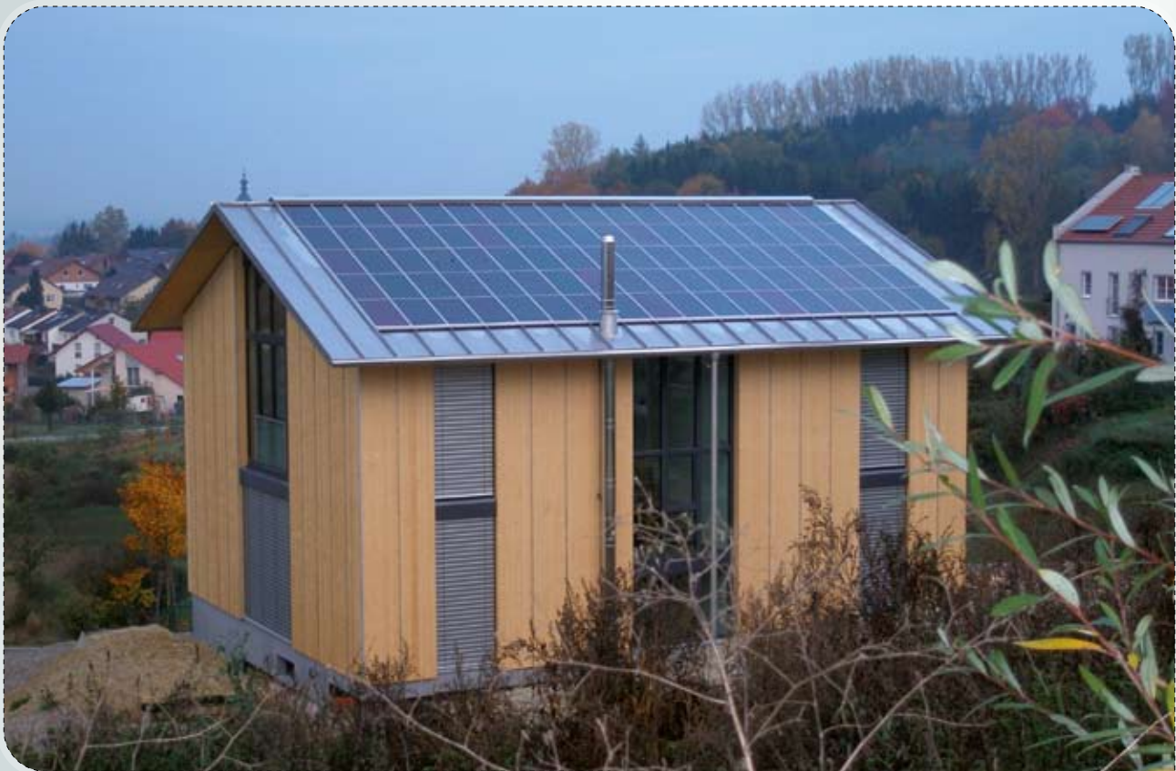
FIGURE 37: Integrated stainless steel and solar technology systems can be applied to buildings of any type and size. (Photo: protectum.de)
