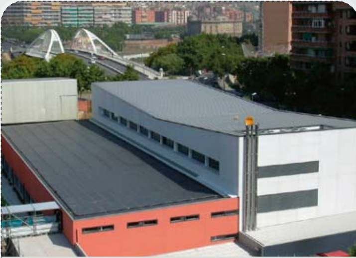
FIGURE 20: The absorbers can fully replace conventional roofing sheet (Photo: energie-solaire.com)
