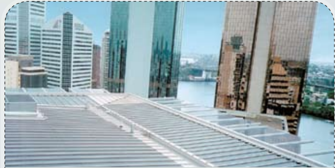
FIGURE 28: Flat stainless steel roof with integrated amorphous PV cells (Photo: uni-solar.com)
