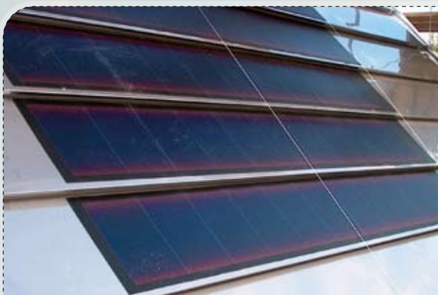
FIGURE 32: Detailed view of a tilted stainless steel roof. Active PV sections can easily be combined with non-active ones. (Photo: thyssen-solartec.com)
