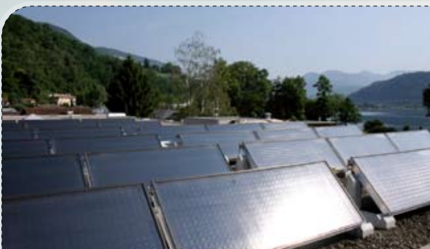
FIGURE 14: Stainless steel cushion-absorbers are a technically and economically favourable option for glazed solar-thermal panels (Photo: energie-solaire.com)
