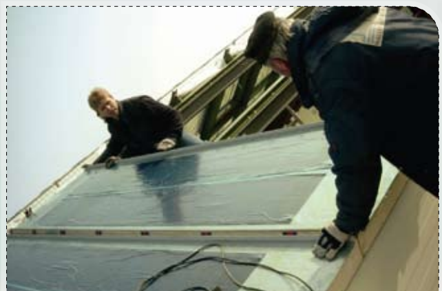
FIGURE 33: Assembly of stainless steel sandwich roofing elements with integrated amorphous PV modules. (Photo: thyssen-solartec.com)
