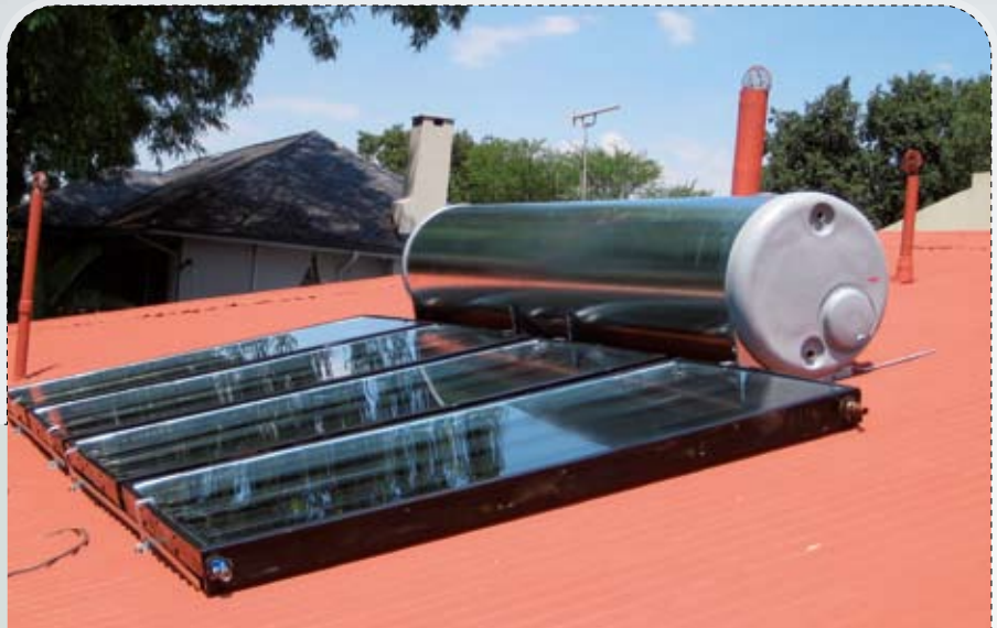
FIGURE 5: Higher-alloyed stainless steel grades are also resistant to coastal atmosphere. The examples shown are situated in locations near the Atlantic coast (Photo: suntank.com)
