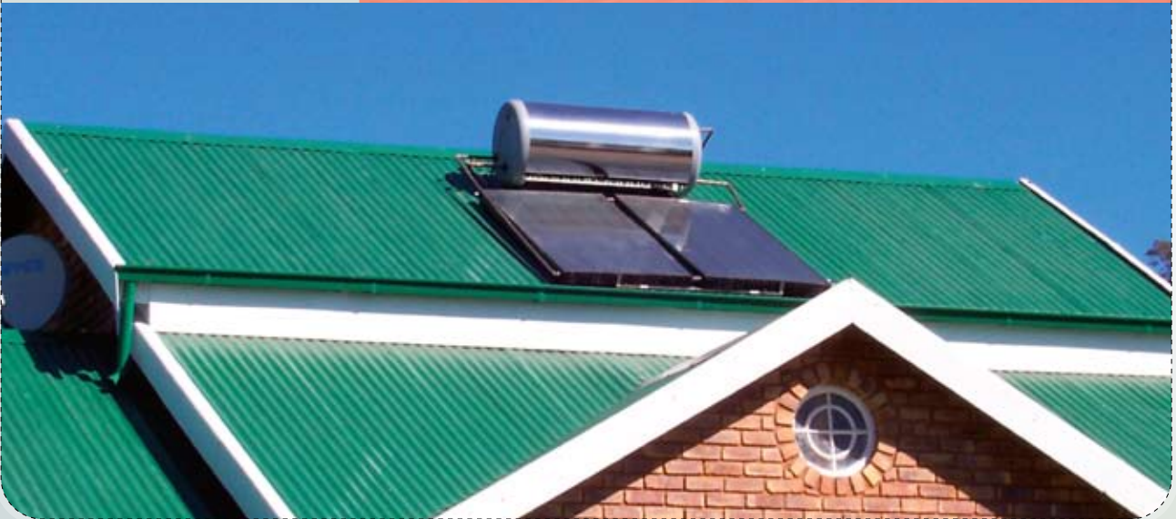
FIGURE 5: Higher-alloyed stainless steel grades are also resistant to coastal atmosphere. The examples shown are situated in locations near the Atlantic coast (Photo: suntank.com)
