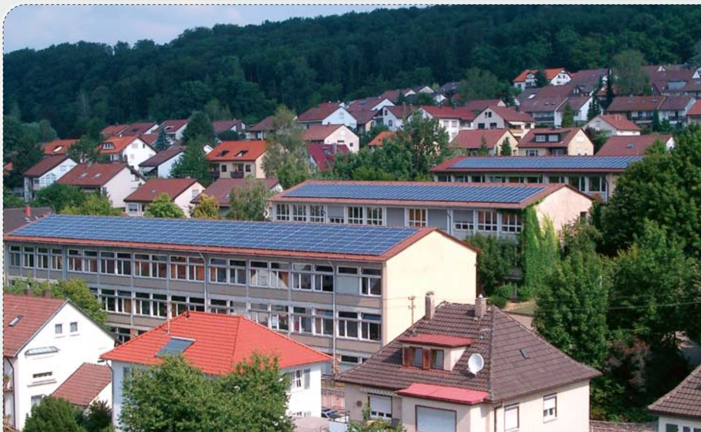
FIGURE 38: PV panels fastened to stainless steel sections (Photo: modersohn.de)
