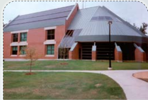
FIGURE 34: Pitched stainless steel roof with integrated amorphous silicon PV modules and non-active parts (Photo: uni-solar.com).
