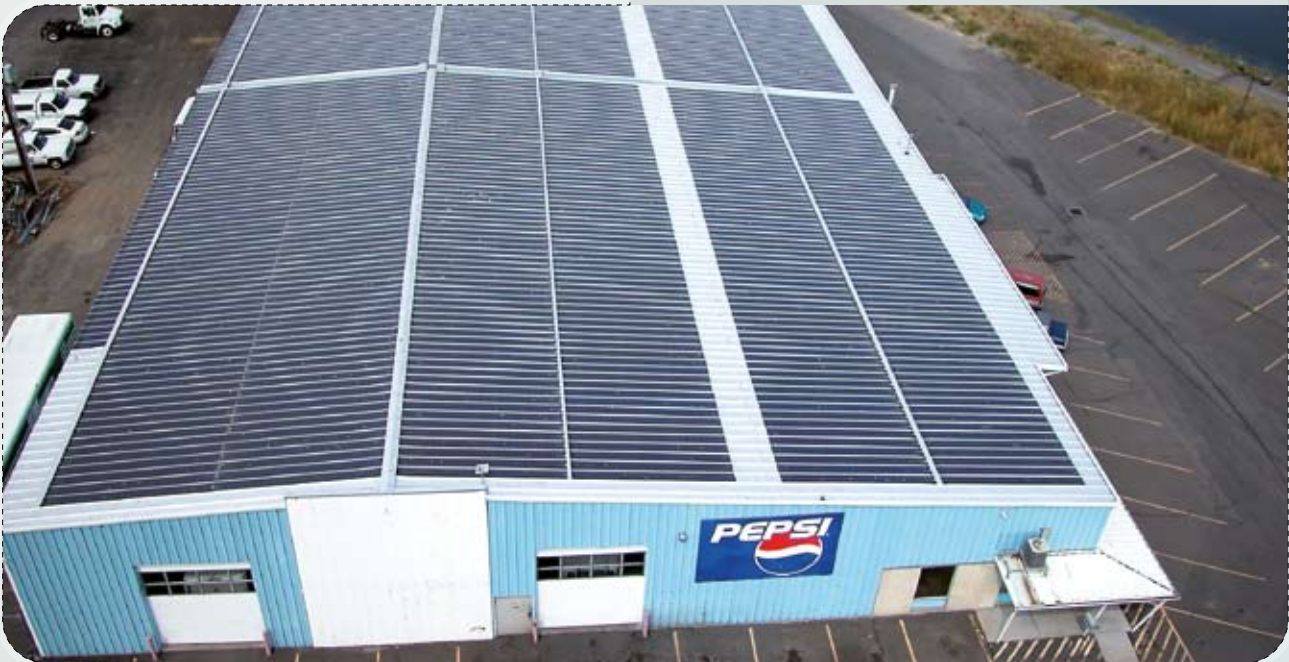
FIGURE 30: Commercial building with a near-flat roof completely covered with multifunctional stainless steel PV units. The electrical output power is about 150 kWh. The annual electrical output in a sunny climate can be up to 300,000 kWh/year. (Photo: uni-solar.com)
