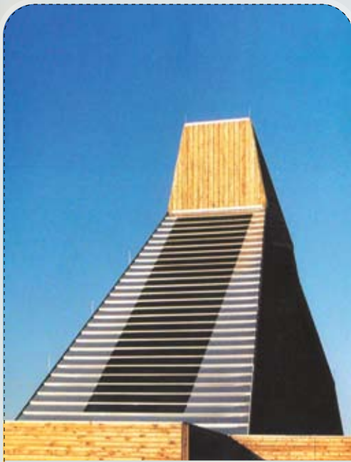
FIGURE 31: The stainless steel tilted roof of a museum building with integrated photovoltaic modules (Photo: thyssen-solartec.com)
