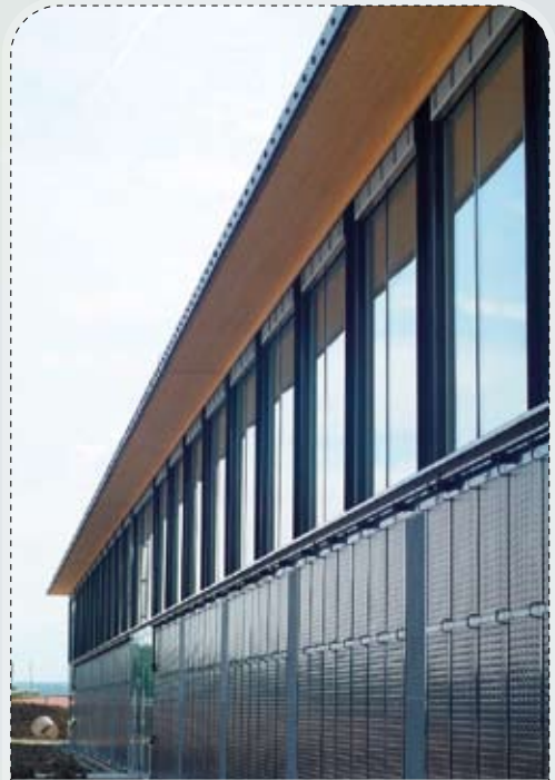
FIGURE 21: The black-chromed surface is efficient as a thermal energy absorber. It blends well with any architectural environment. (Photo: energie-solaire.com)
